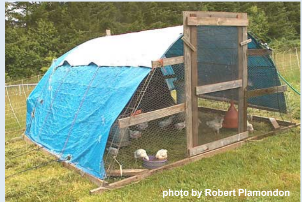
Cattle-panel hoophouse. The front and back walls are framed with 1x4 lumber and covered with chicken wire. The door is a hatch that lifts out.
