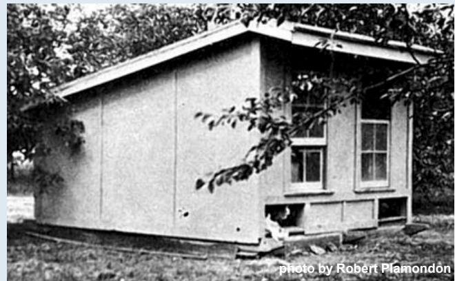
Traditional all-season colony house used in the past. For extra ventilation in summer, the window sashes are removed and a full-width vent in back is opened under the eaves.
